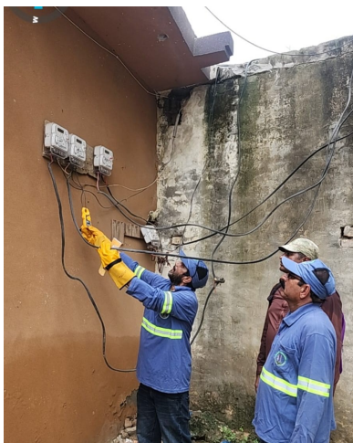
(b) LESCO staff testing consumer meters during a combing visit, Combing arm, August 2026.
